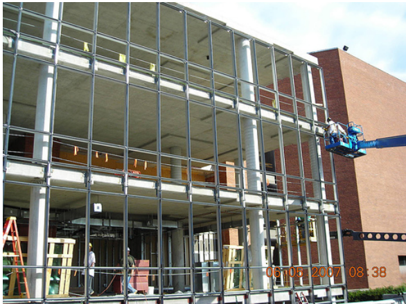
Fig. 1: Applying aluminum grid around addition perimeter
