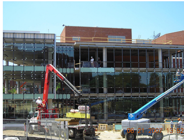
Fig. 2: Two genies erecting glass
