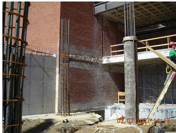
Fig. 5: Pouring columns in lower level addition
