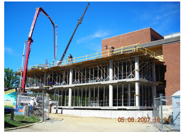
Fig. 6: Pouring slabs with truck and pump
