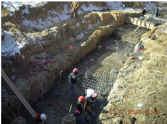
Fig. 4: Pouring footings along curved foundation wall
