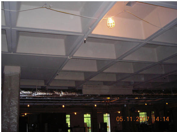
Fig. 7: Insulating duct work & painting existing waffle slab on first floor
