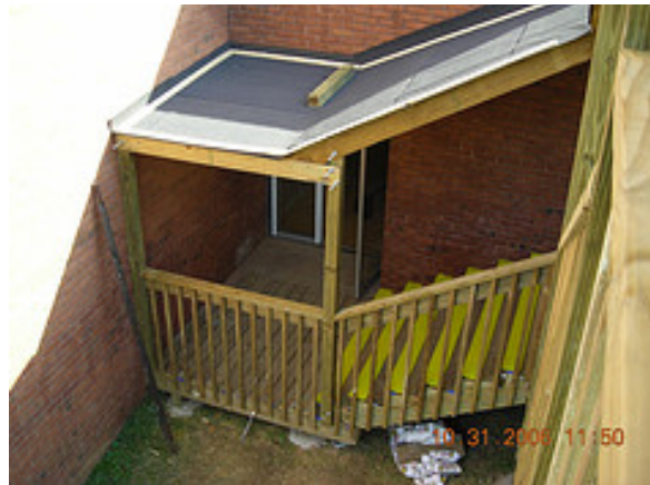
Fig. 2: Temporary steps for public access to library at west entrance
