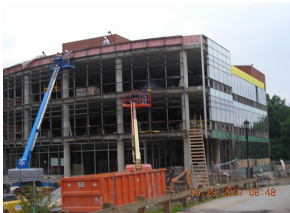
Fig. 4: More glass and insulation installation
