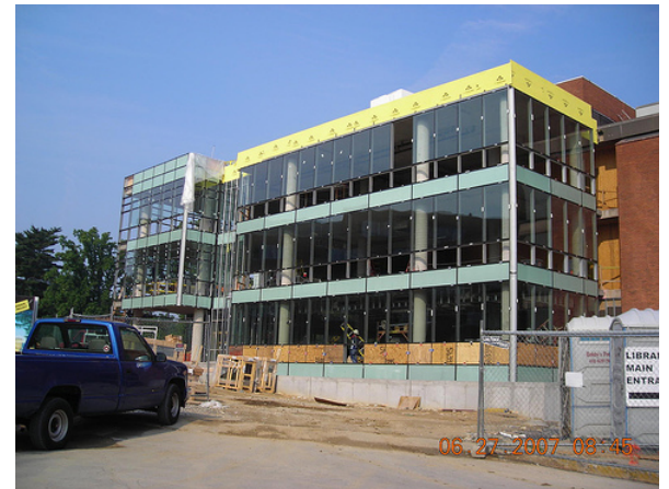
Fig. 3: Applying insulation at top of third floor
