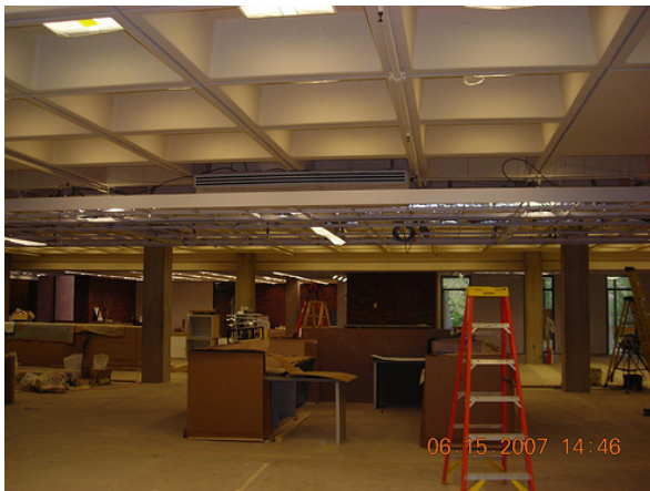
Fig. 10: Hanging of Floating Ceiling
