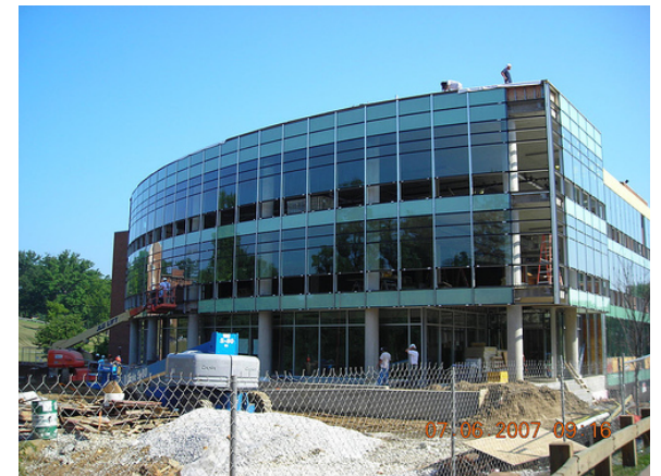
Fig. 6: New addition curtain wall 85% complete
