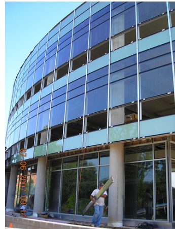
Fig. 5: Close Up after installation of clear and spandrel glass
