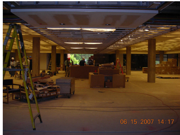
Fig. 8: Installing light fixtures
