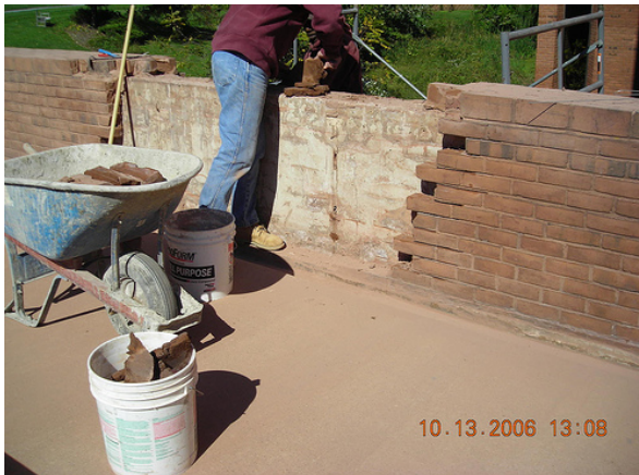
Fig. 1: Removal of wall and steps
